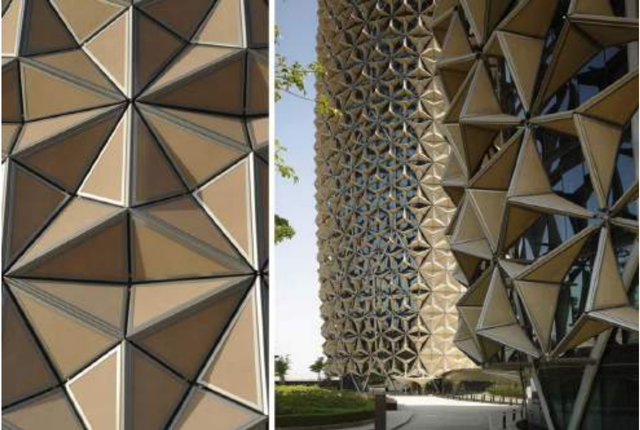
Al Bahar Tower Abu Dhabi Highlighting Responsive Façade
